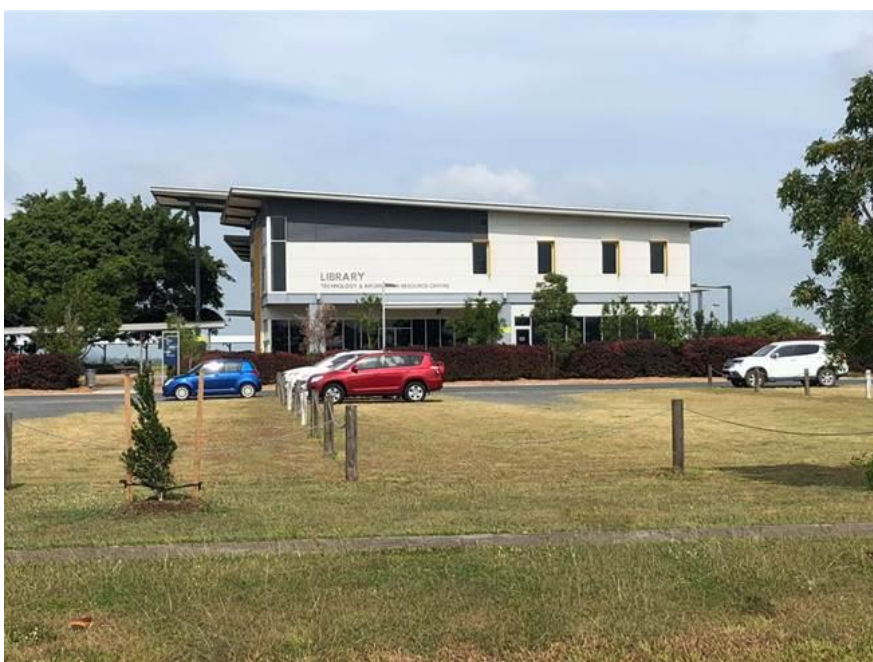
Photo taken from East end of Library building.
